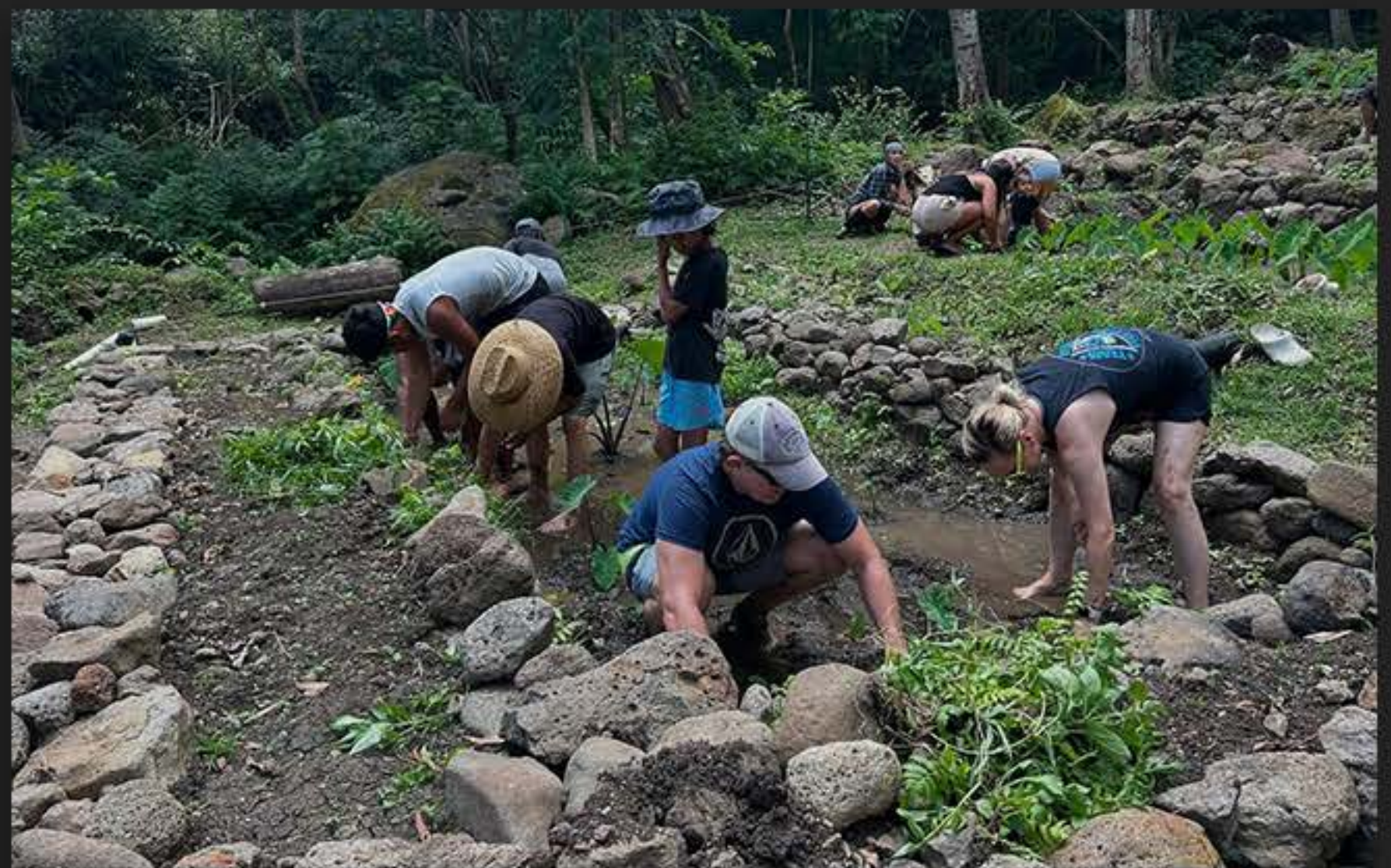
Nation of Hawaii members show the progress of their work in 2024 to build a rock wall for capturing water for a traditional taro bed on their land in Pu'uhonua village, Oahu.
